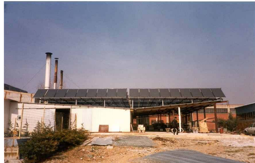
Selective flat plate collectors on roof
