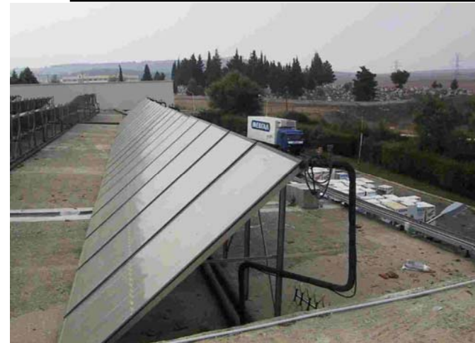
Selective flat plate collectors on roof
