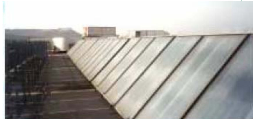
Selective flat plate collectors on roof
